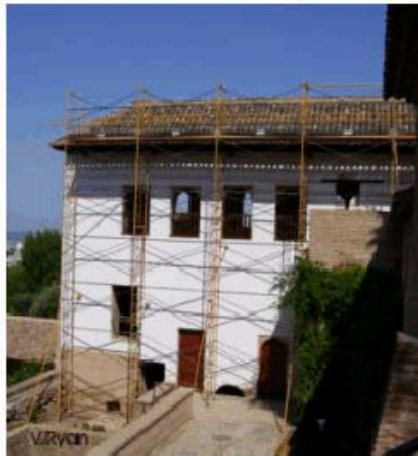
SCAFFOLDING FOR A BUILDING
