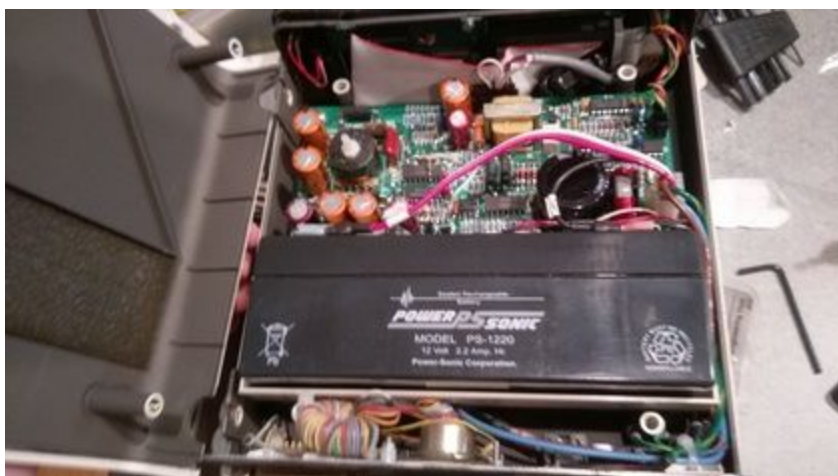
The first view upon removing the top lid.
