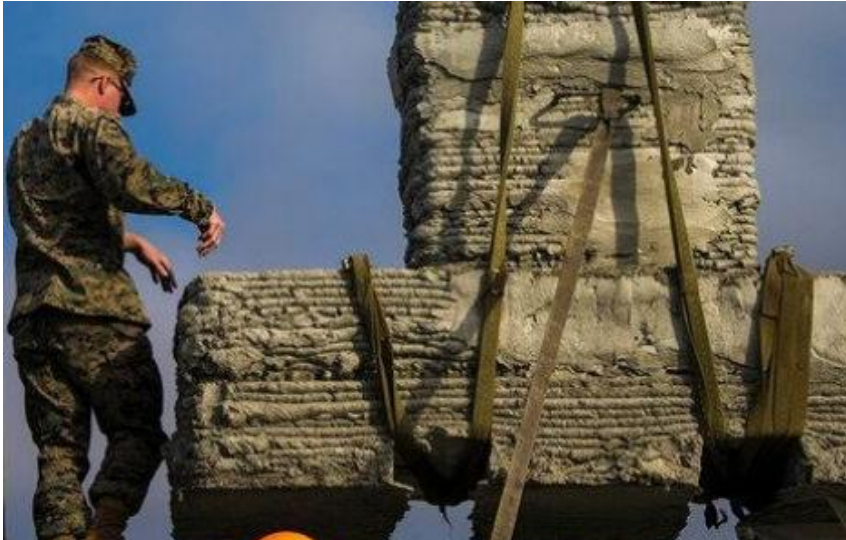
13 Securing a 3D Concrete Bridge Support ( https://www.foxnews.com/tech/marines-3d-print-amazing-concrete-bridge )
