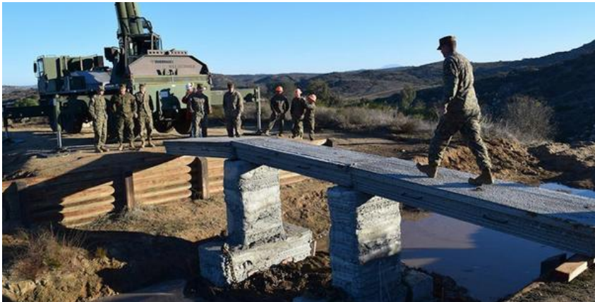
14 3D Concrete Printed Foot Bridge ( https://www.military.com/dodbuzz.com/dodbuzz/2019/01/31/marines-just-3d-printed-entire-bridge-california.html )
