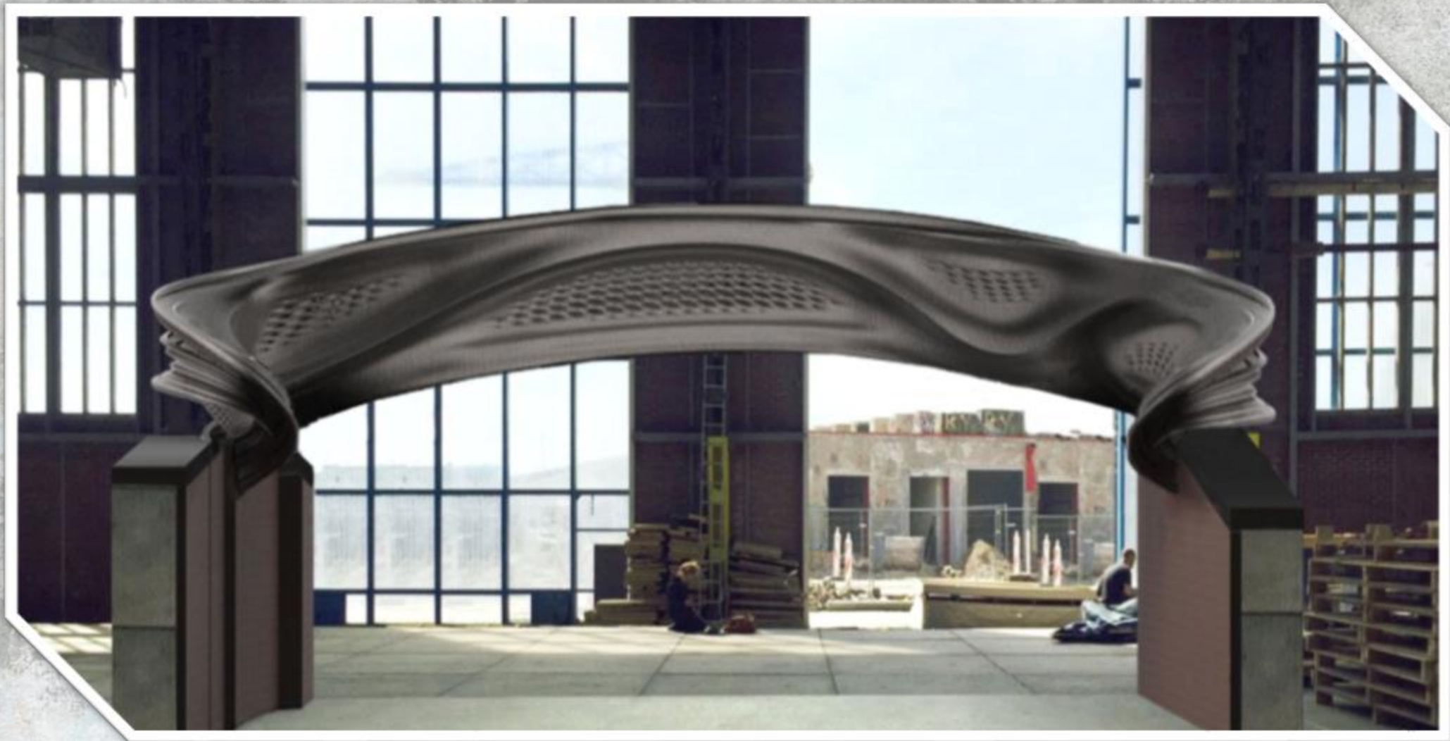
12 Finished Amsterdam Steel Pedestrian Bridge Before Being Put in Place ( https://www.jorislaarmaPcom/work/bridge-update )
