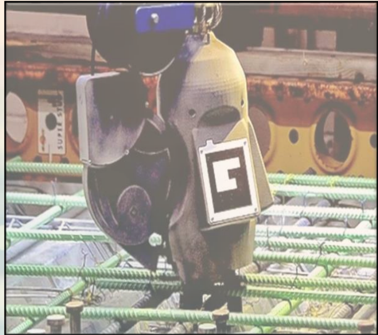
5 TyBot Tying Rebar ( https://www.tybotllc.com/get-tybot )
