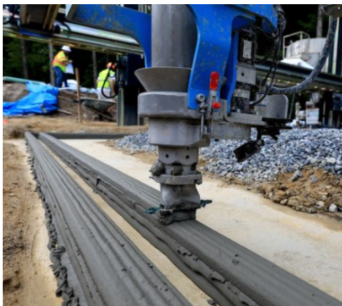
Alquist 3D printing process using concrete layers (Alquist)
