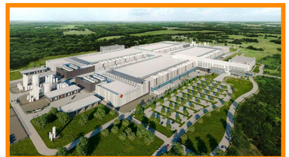
Manufacturing Site in Sherman, Texas.
