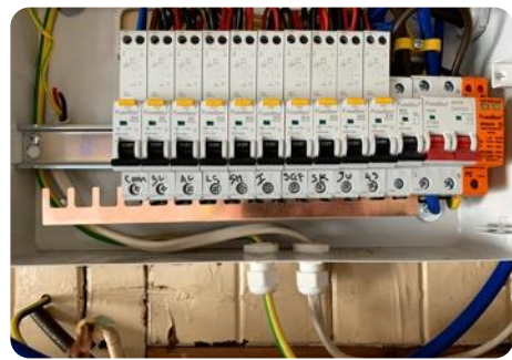
Fig 1.3, A generic, British consumer unit fitted with RCBO's (Single Phase.)
