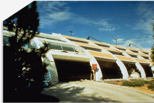
Collapse of concrete parking structures during 1994 Northridge Earthquake
