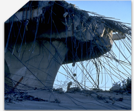
Failed support columns from 1994 Northridge Earthquake
