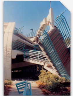
Collapse of concrete parking structures during 1994 Northridge Earthquake
