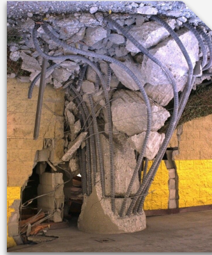
Failed support columns from 1994 Northridge Earthquake
